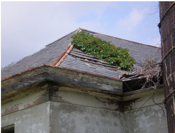
Figure 4-1: Front room roof
