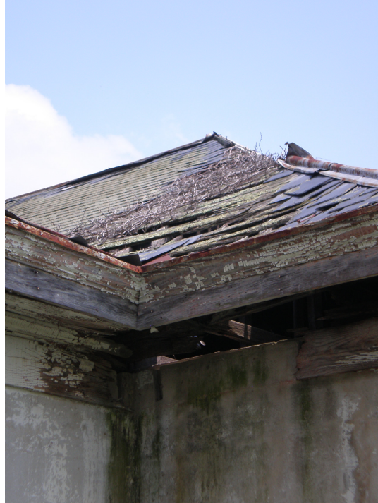
Figure 4-3: Gutter deterioration
