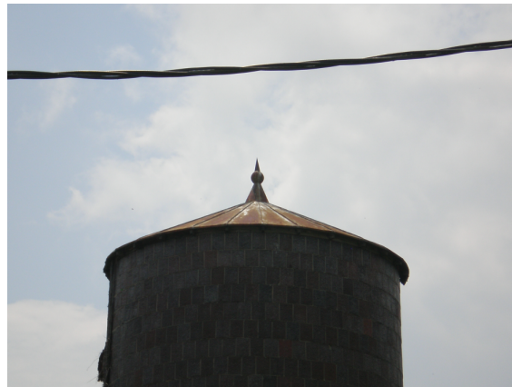
Figure 2-9: Current silo roofs
