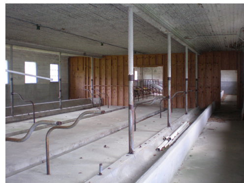
Figure 2-6: Wait Station/Feeding Room
