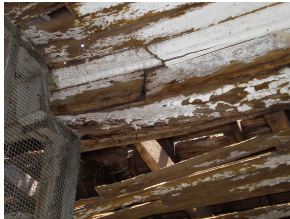
Figure 4-2: Front room ceiling
