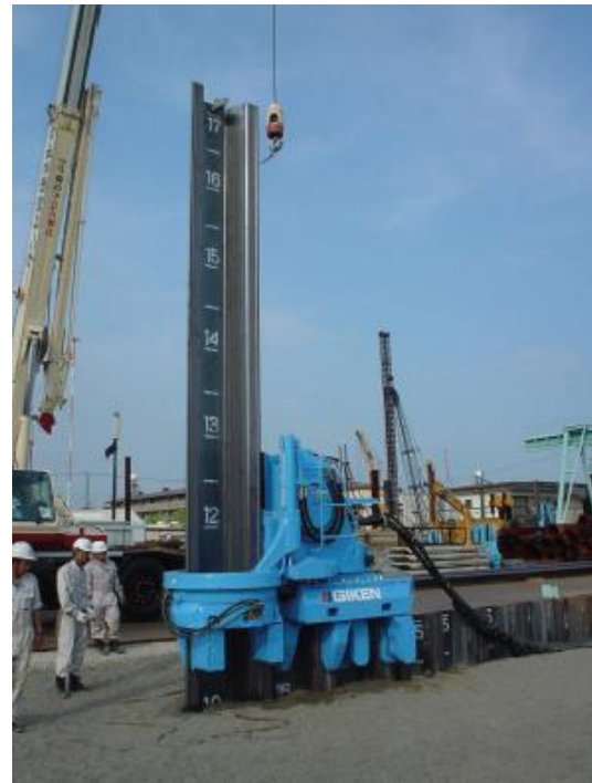
Figure6b: Hydraulic jacking Method
