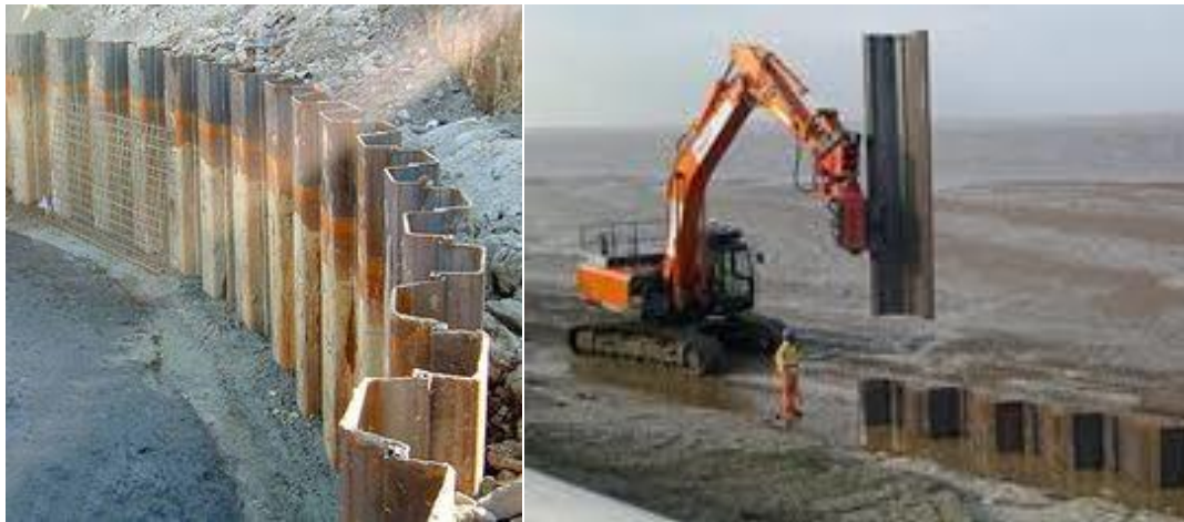
FIGURE 1: SHEET PILING WALL (DESIGNBUILDINGS, 2017)
