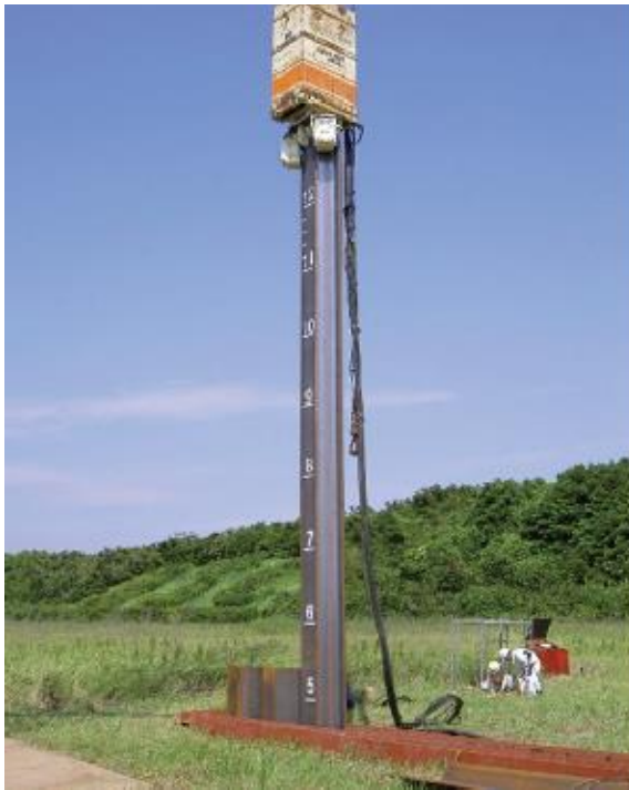
Figure6a: Vibratory Driving Method
