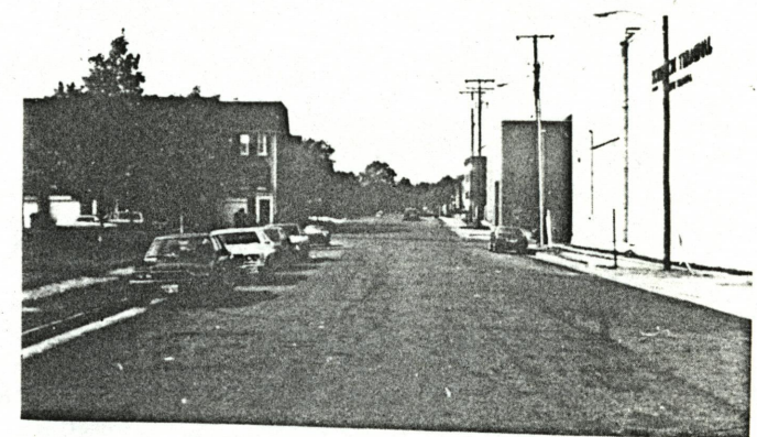
Oronoco Street looking West, Robinson Terminal on the right
