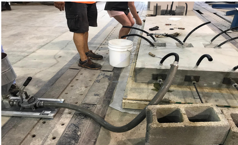
Figure 3-8 Grouting Process
