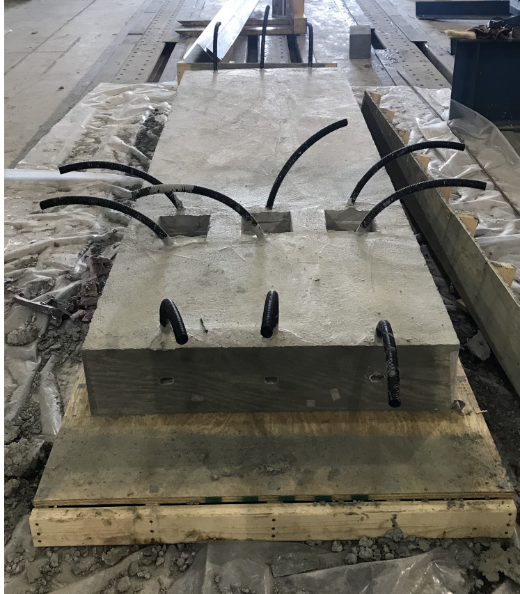
Figure 3-6 The Slab After Concrete was Placed
