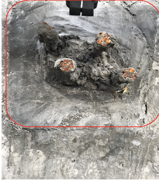
Figure 3-22 The Pour-Back Material in the Block Out Pockets
