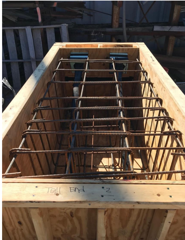
Figure 3-18 Reinforcement at the End Section
