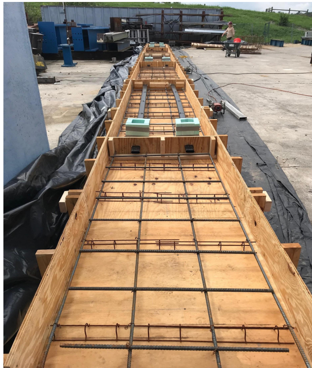
Figure 3-17 Transverse and Longitudinal Reinforcement and the Ducts
