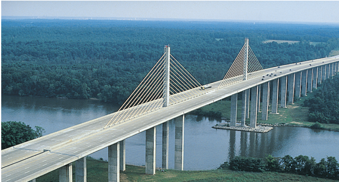
Figure 1-1 The Varina-Enon Bridge (Figg, 2019)
