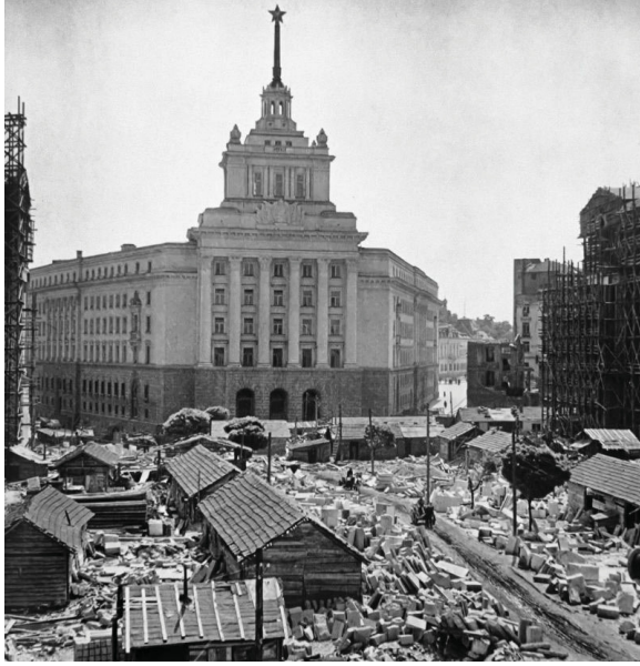
Fig. 1. Downtown Sofia in the 1950s. The newly built House of the Communist Party towers above some shabby homes soon to be demolished for a large ceremonial plaza (the Largo). Such ceremonial plazas were a spatial hallmark of socialist regimes and were meant to convey their triumph over petty private interests. Source: http://www.stara-sofia.com
