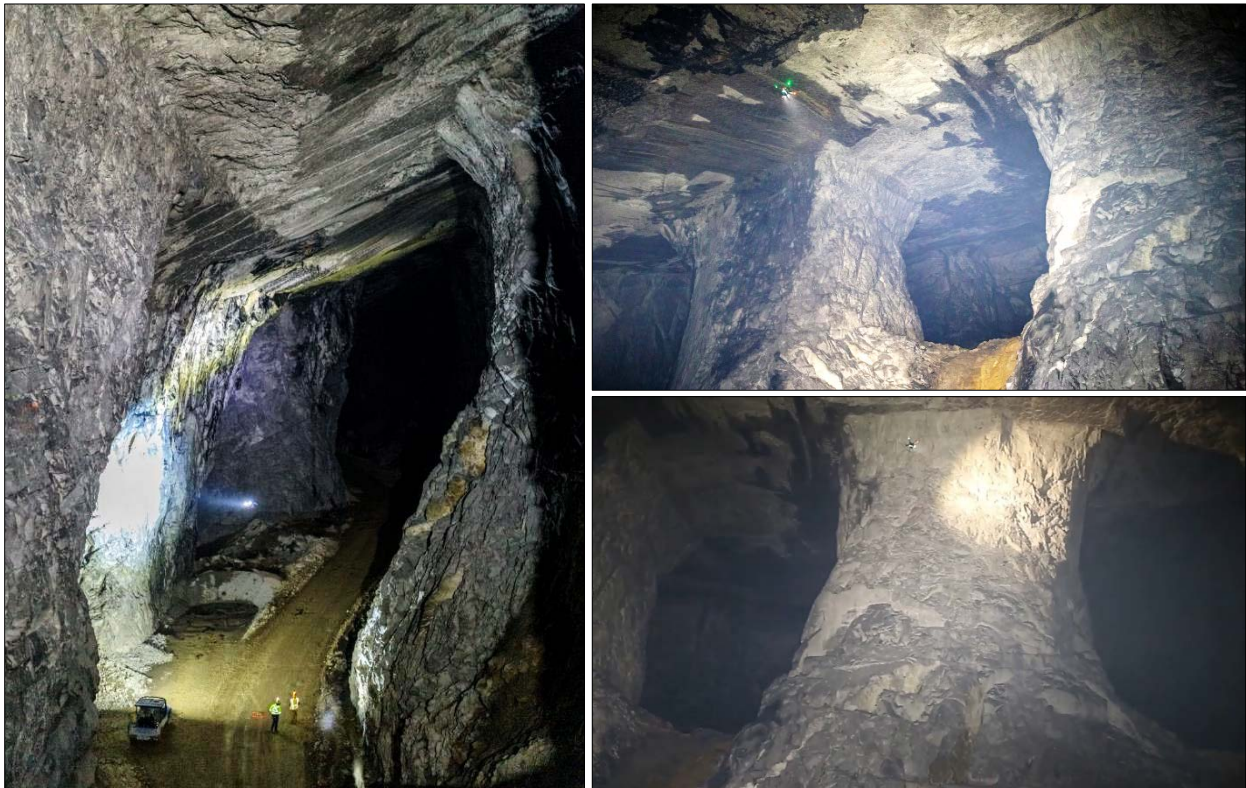
Figure 4.10 LiDAR and Photogrammetric surveys around Pillar B. The picture on the left shows the drone able to map inaccessible heights around the pillar [16].
