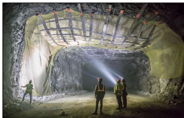
Fig. 4 Ground support around Pillar-X (Credits: R. Bishop)
