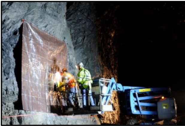
Fig. 5 3D GPR survey conducted along the Pillar-X
