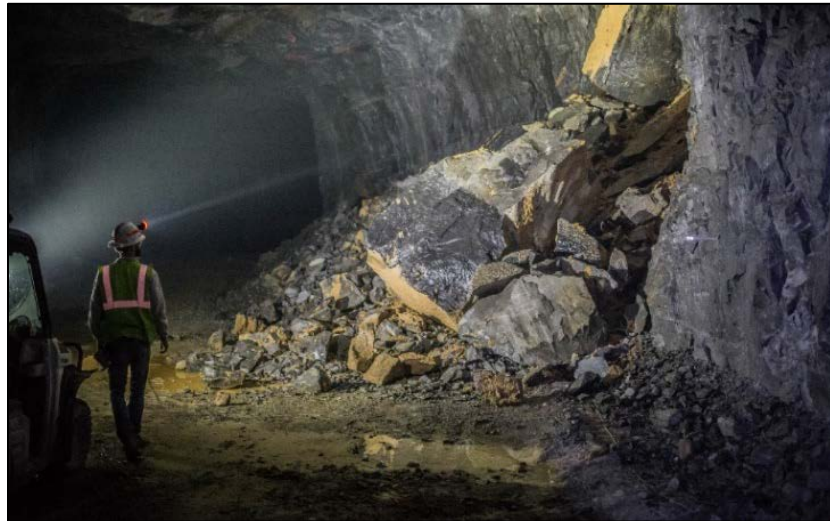
Figure 2.3 Material collapse from karst void in the case study mine [18].
