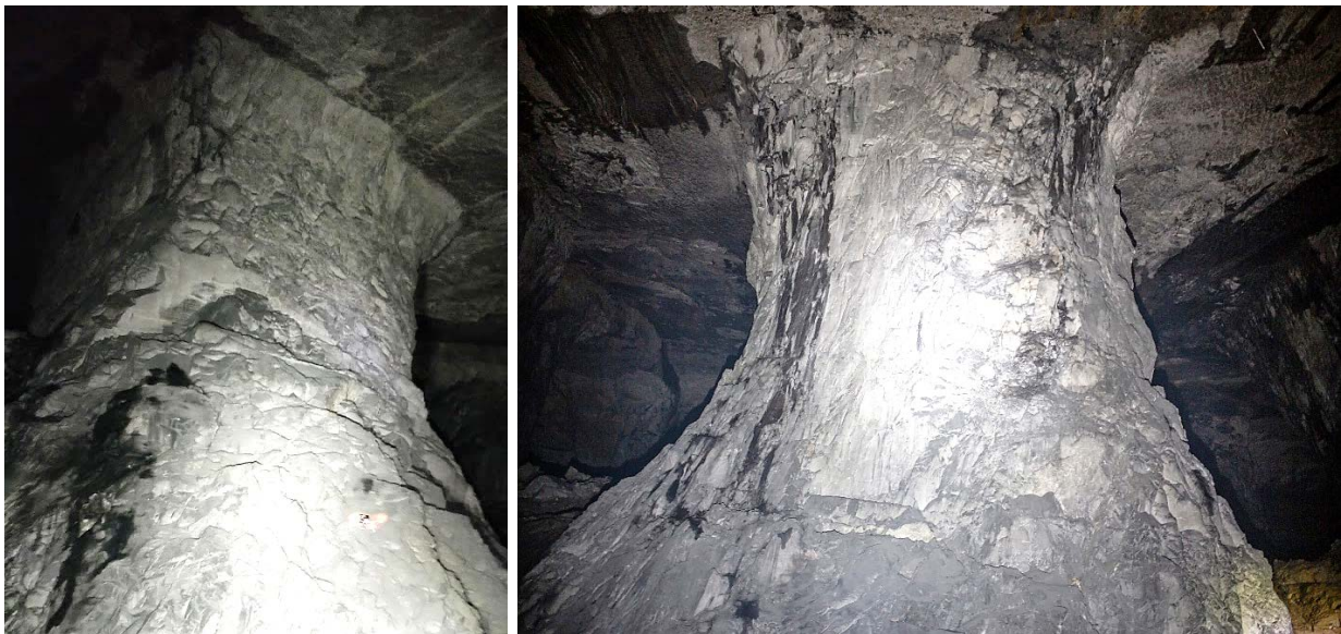
Figure 6.1 Tall, inclined pillars in the case study mine.
