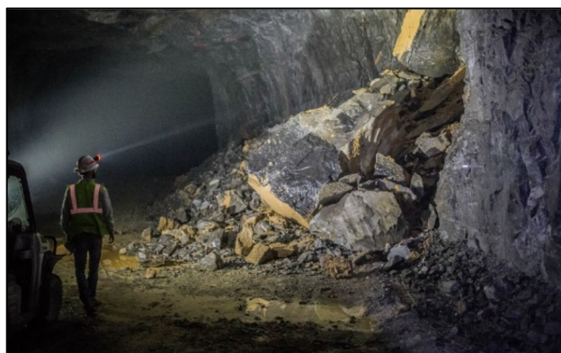
Fig. 3 Material collapse from karst void in the case study mine (Credits: R. Bishop)
