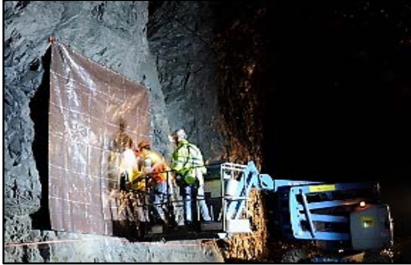
Figure 2.5 3D GPR survey conducted along the Pillar-X.
