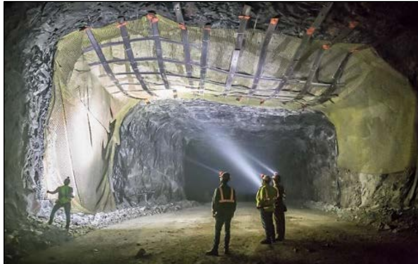
Figure 2.4 Ground support around Pillar-X [18].
