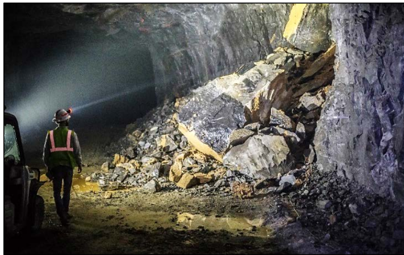
Figure 5.2 Ground failure caused due to collapse of karst void [18].
