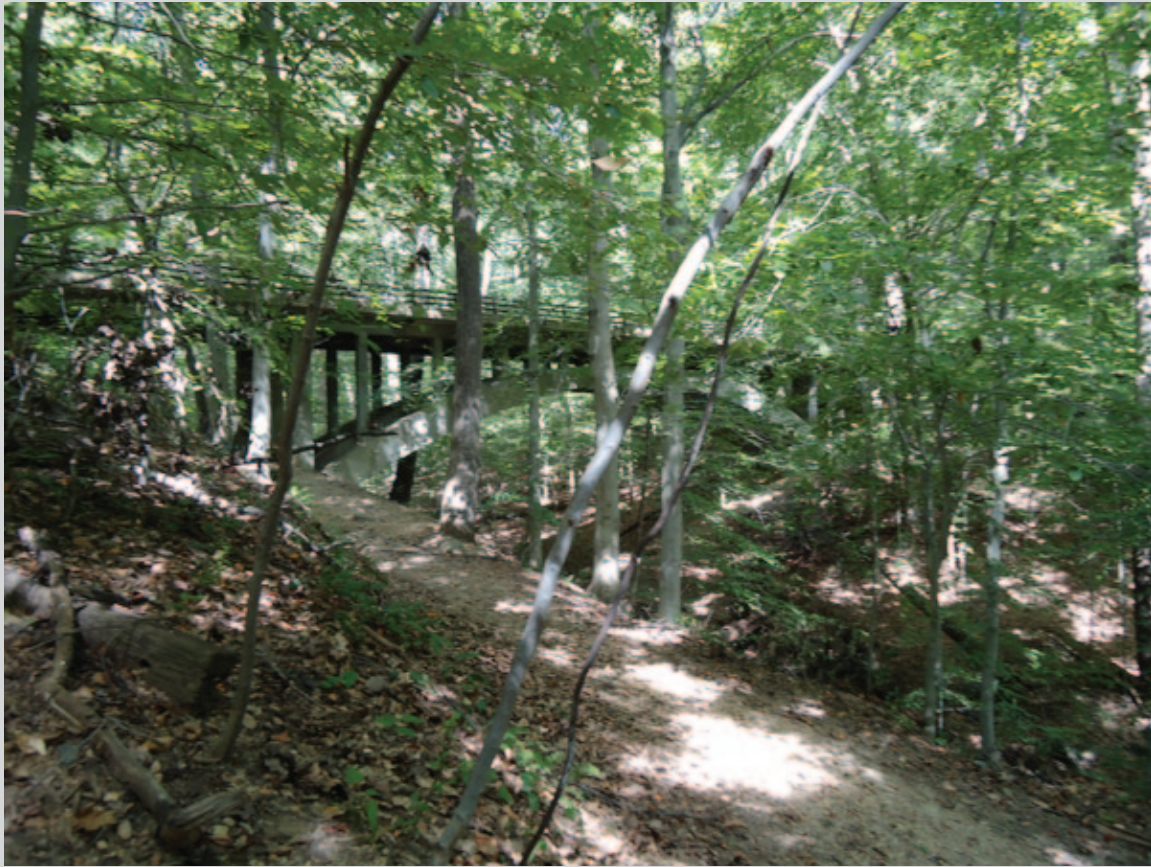
Site photo looking north toward Ridge Road bridge
