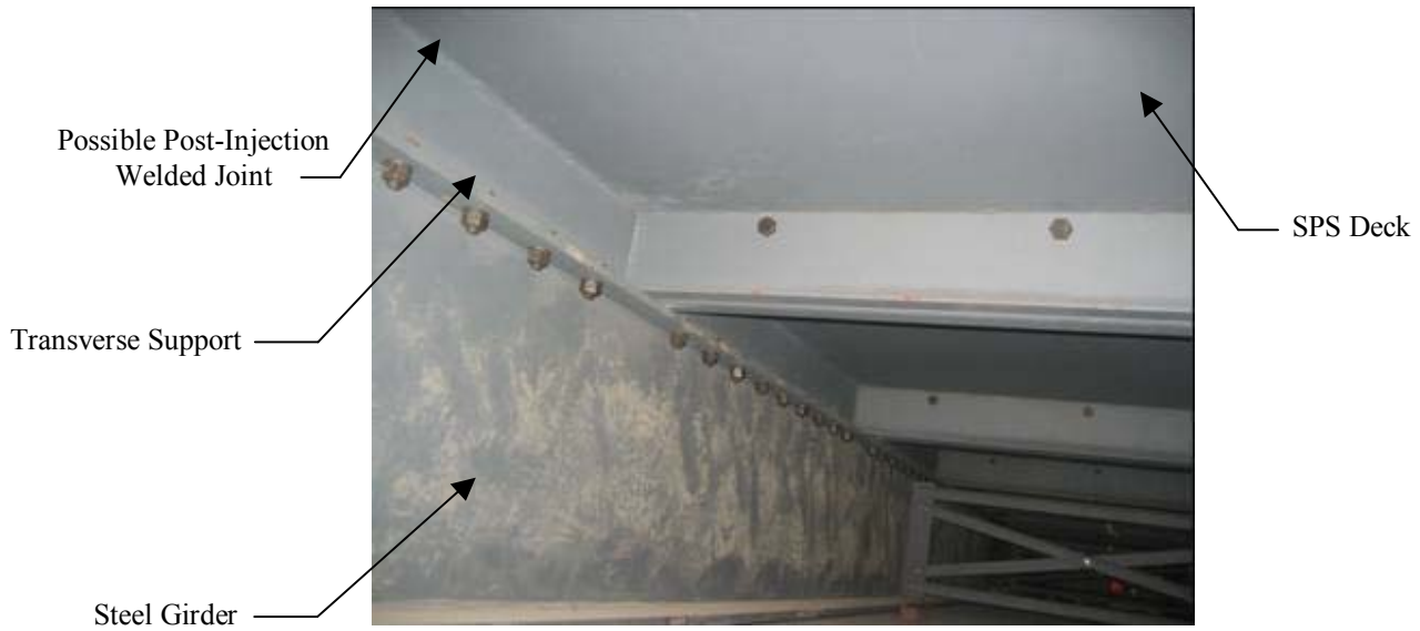
Figure 1.4 Transverse support welded to SPS deck and steel girder.
