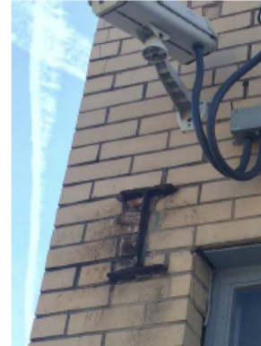
Exposed steel beam
