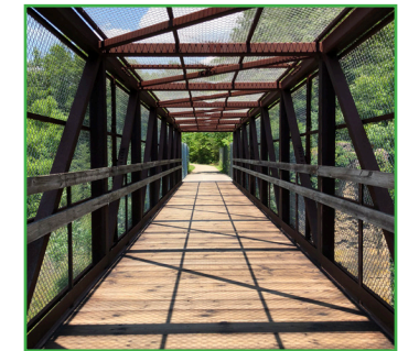
Fig.34: Pedestrian bridge along the trail
