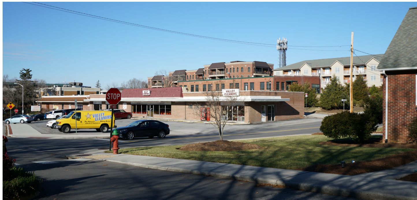
Fig.11: View of Daper Road Mini-Mall, the site, from low density residential neighborhood with peripheral commercial downtown and civic buildings
