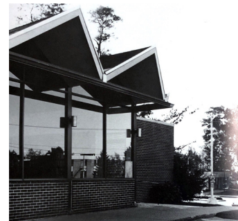
Fig.29: Folded roof, former public library building
