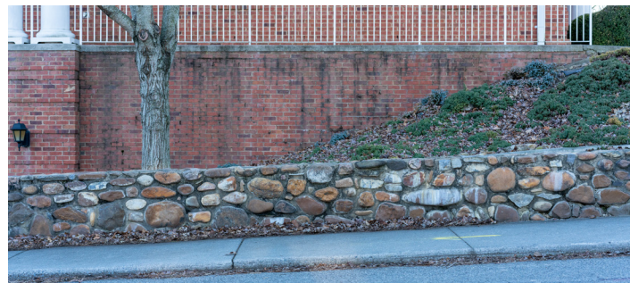
Fig.15: Exemplary Blacksburg retaining wall
