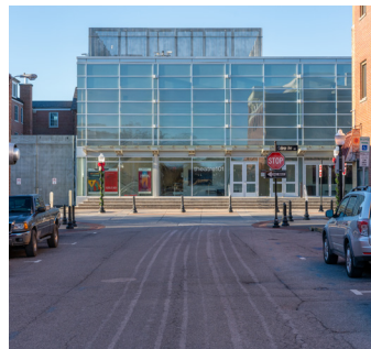
Fig.14: Theatre 101 at termination of Draper Rd
