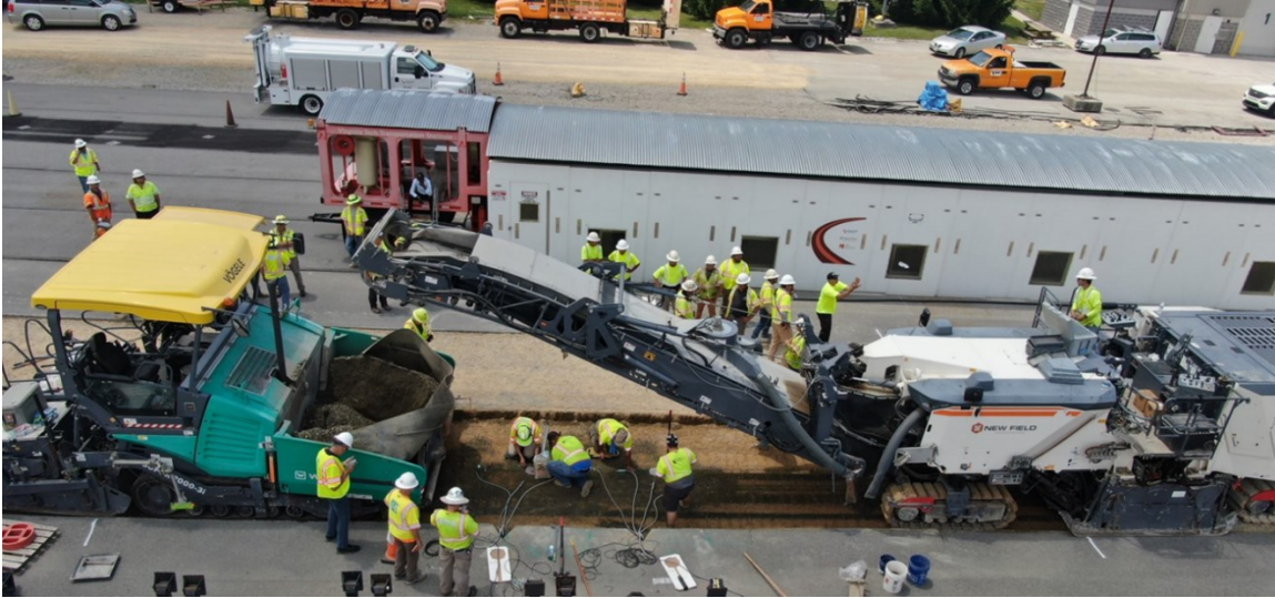
Figure 2-6 1 . Virginia APT facility and field construction at VTTI.
