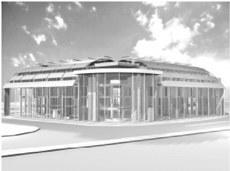
southeast corner view (transparency of the corner)
