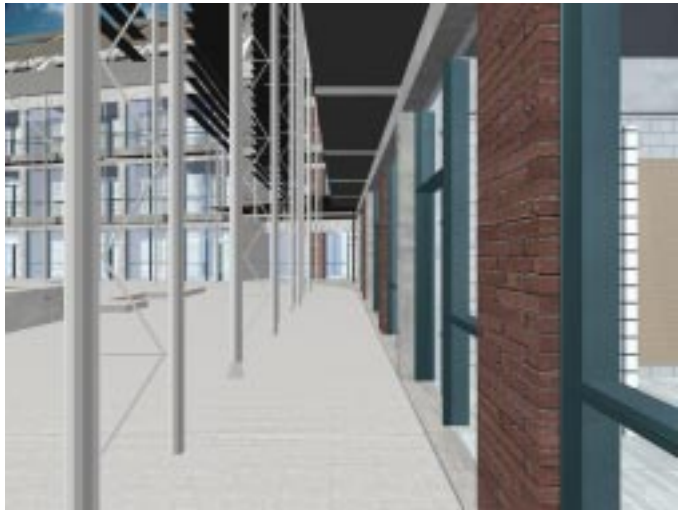
glass wall enclosing the shop and steel columns and shades
