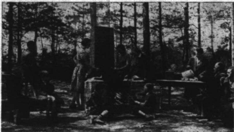
Well-built, but firebox should be raised nearer cooking surface.
