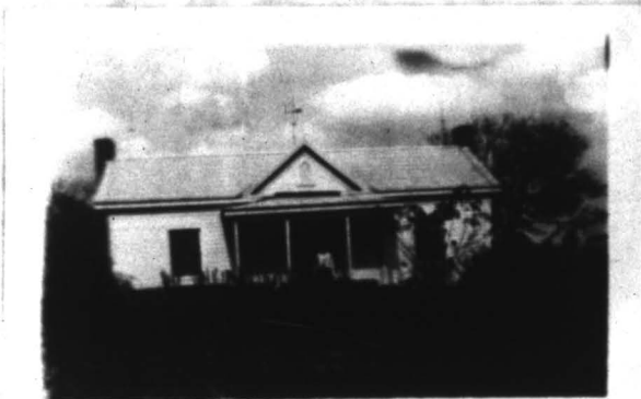
A demonstration community activity. Repainted home of Tim Robinson, R #1, Pleasant Hill, N. C., Dahlia Community.
