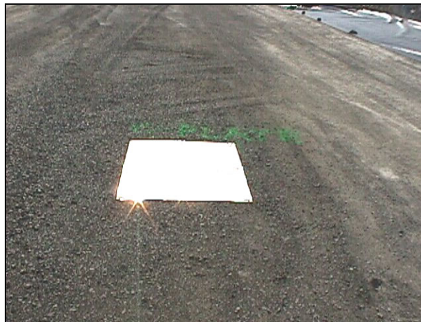
Figure 3-1: Copper plate under 21-B material in section B
