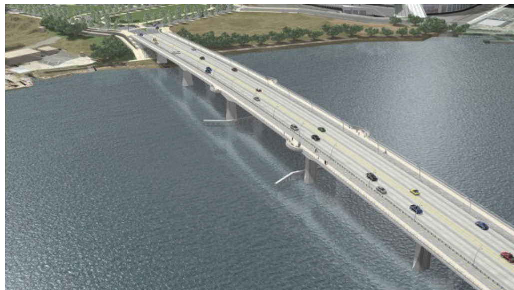
12. New Frederick Douglass Memorial Bridge
