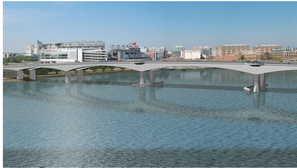
10. New Frederick Douglass Memorial Bridge
