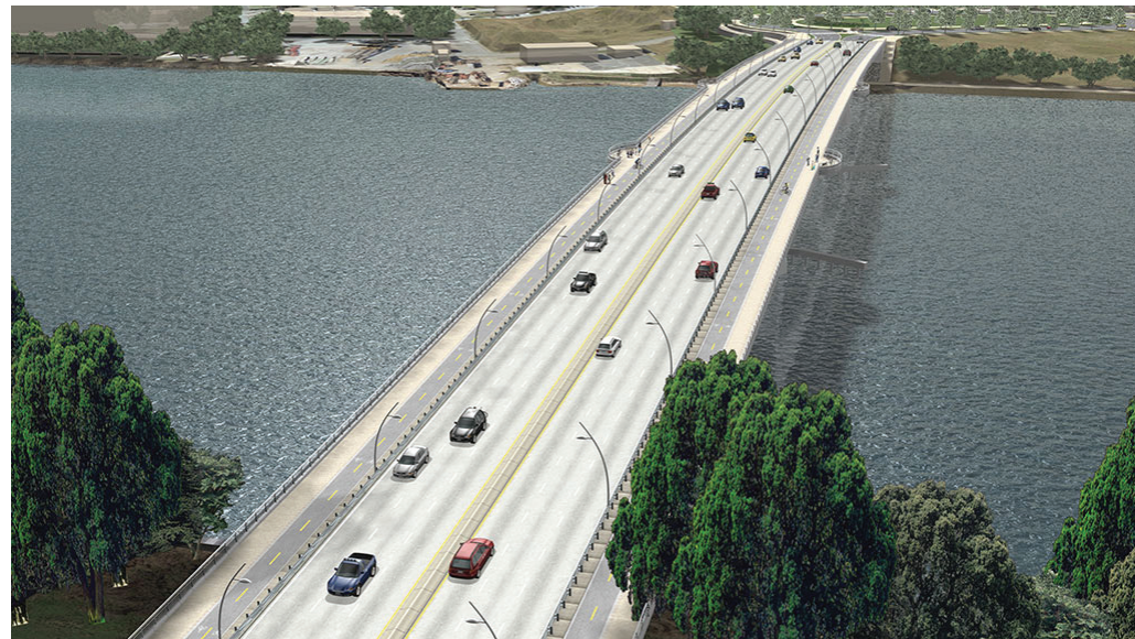
11. New Frederick Douglass Memorial Bridge
