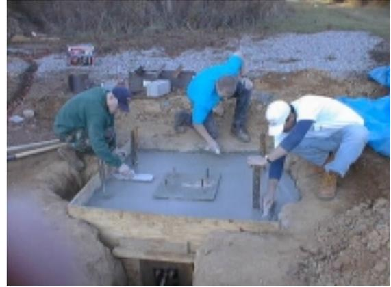
(b) Finishing concrete surface of 36" deep cap.
