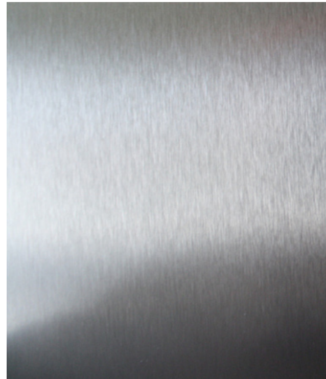
FIG 77 - PHOTOGRAPH WEATHERED STEEL
