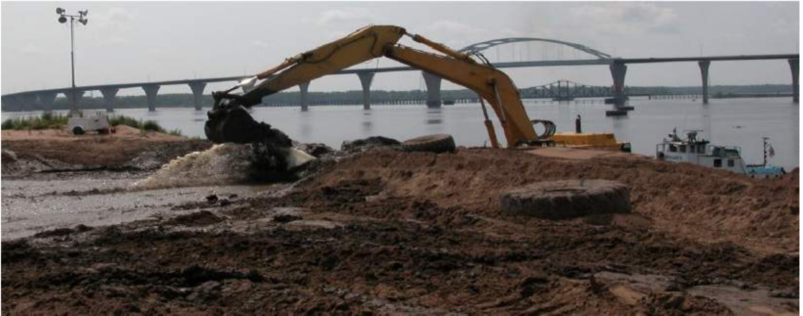
Erie Pier - Mechanical offloading of dredge
