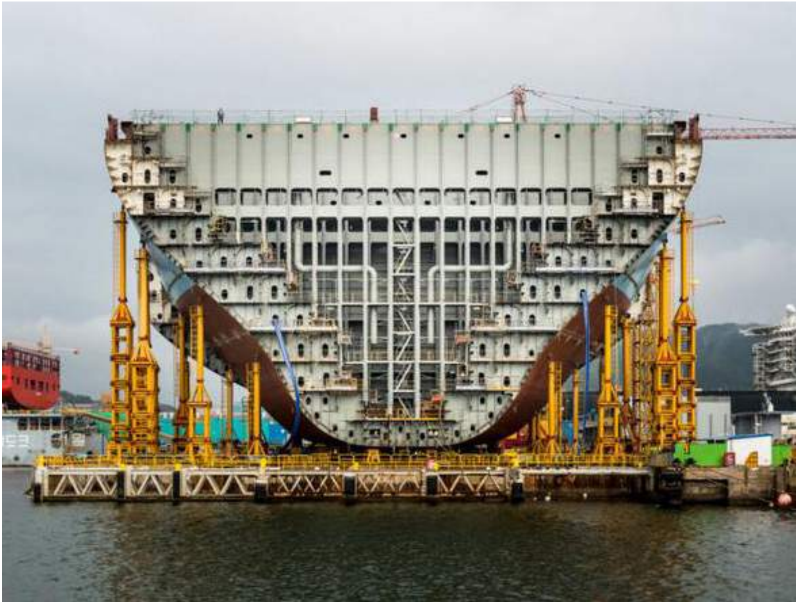
Sectional View of Maersk Triple E Class under construction
