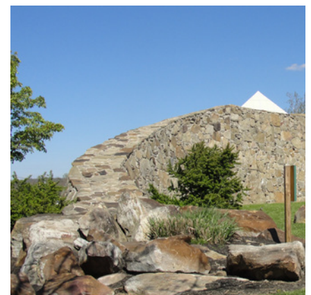
Stone reflects highway noise away from grounds
