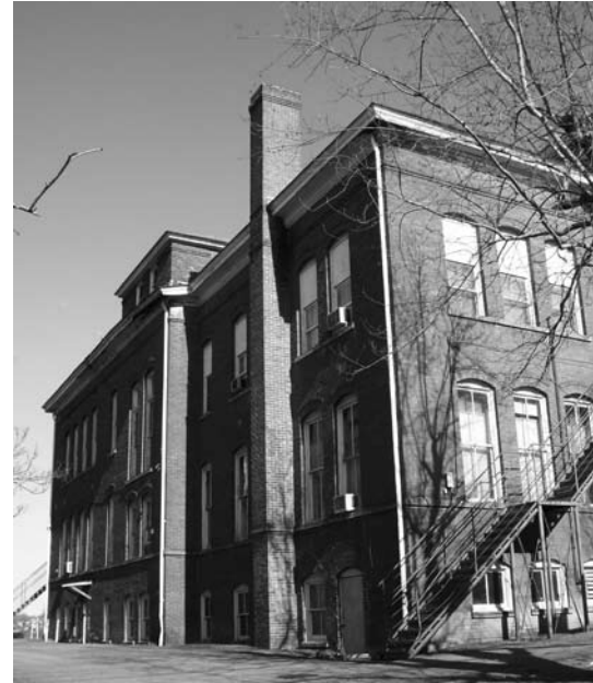
view at northwest corner
