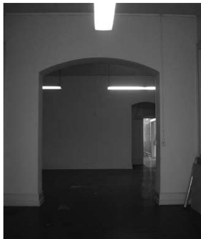
view of arched opening from west corridor
