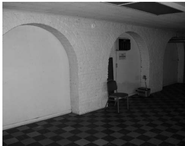
masonry arches in existing basement
