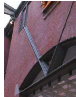
Figure 4.5. Steel beams imbedded in the brick atrium walls of the Holocaust Museum.
