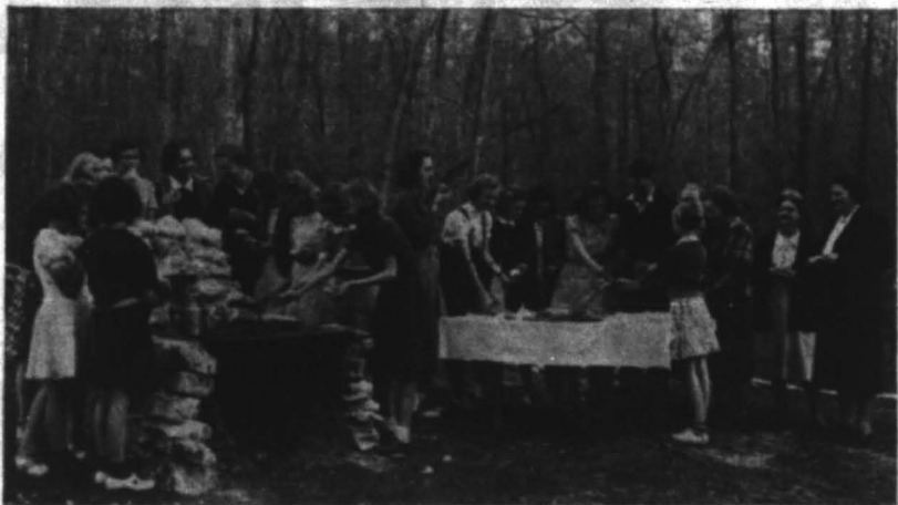
Attractive spot, but firebox much too big. Firebox may be raised by putting loose stones in the bottom. Cooking surface low even for children.
