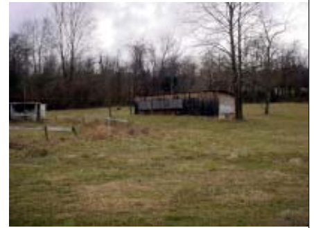
View of existing horse barn and arena
