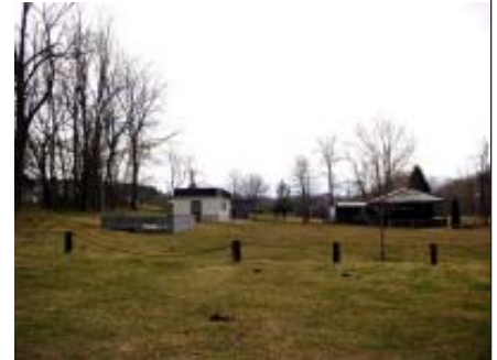
(L to R) Restroom foundation, concession building (white), and bandstand on western 1/2 of site
