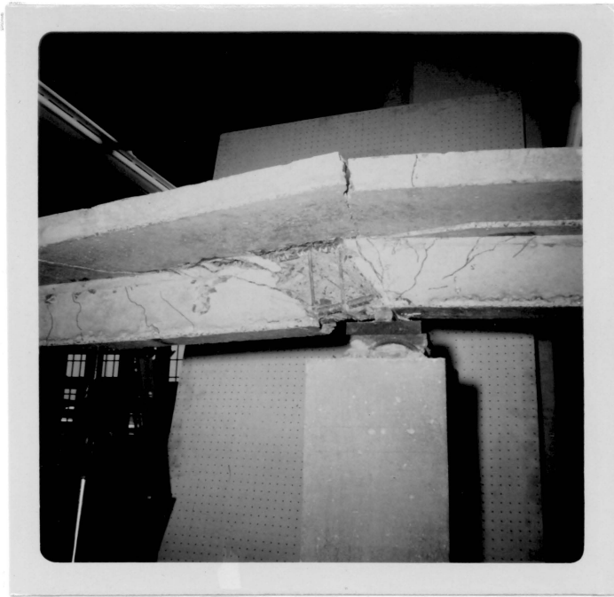
Figure 13. Appearance of Failed Support Section, Beam No. 2
