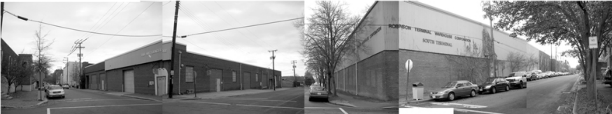
Photo B. Panoramic photo montage of industrial brick and corrugated metal buildings. View straight ahead is towards Duke Street's dead end at the Potomac's river front.
