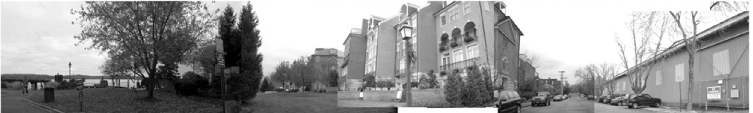
Photo C. Panoramic photo montage of Potomac River front with fragmented bike path, new townhomes with green space, Wolfe Street, and project site on right.
