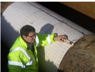
Figure 2-15: BEM Hand-Held Tool Being Used to Scan a Gray Cast Iron Pipe. (WRF, 2008)
