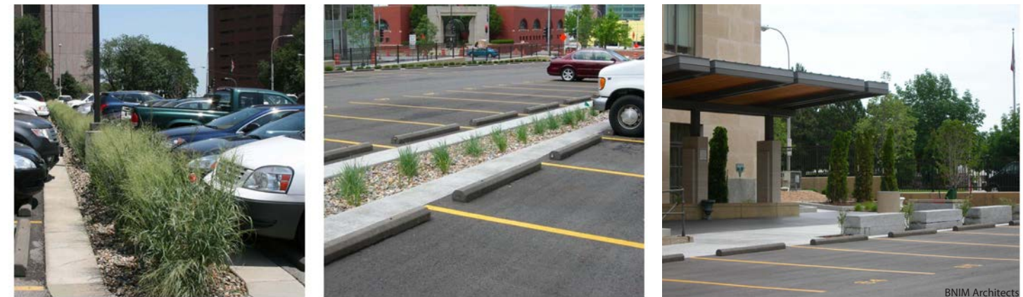
In 2005 BNIM Architects designed a green parking lot that uses bioswales to collect and filter stormwater from the surrounding paved area and courthouse roof. Flat curbs were used throughout the lot to allow water to flow off of the paved surface and into the bioswales. The wheel stops selected for the lot are made with 100% recycled plastic.
