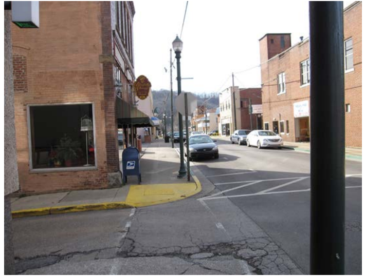
Narrow sidewalks, overhead line, and storefront awnings limit the location and type of street trees that can be planted along Main Street.
