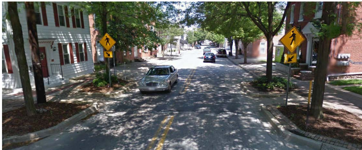
Curb extensions create more room for larger street tree planters. Large planters provide more room for roots to grow, resulting in healthier trees and a more comfortable, shaded street.
