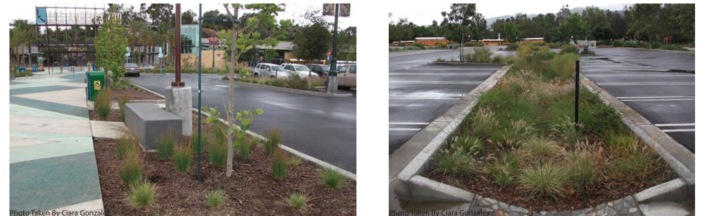
In 2011 the Log Angeles Zoo parking lot was constructed to mimic natural hydrology and reduce storm runoff. A combination of permeable paving and bioswales slow and capture stormwater where it infiltrates into the ground near its point of impact. The large parking lot was planted with 247 trees, nearly four times as many as it had before reconstruction. The trees are located and planted in a way that provides as much shade as possible, reducing the heat island effect created by direct sunlight shining on paved surfaces.
