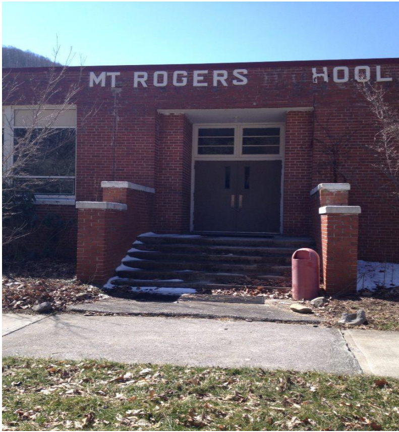
Main entrance of the school, Spring 2013
