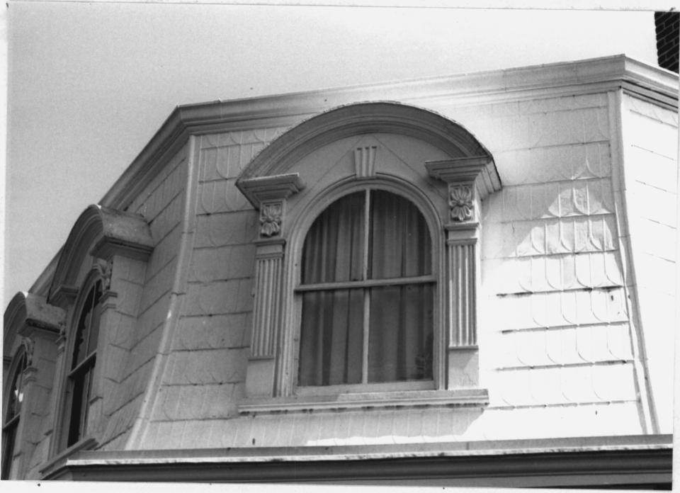
Fig. 12. Full third floor and mansard roof of Preston Hall following 1905 renovation. Photograph by G. Hall
