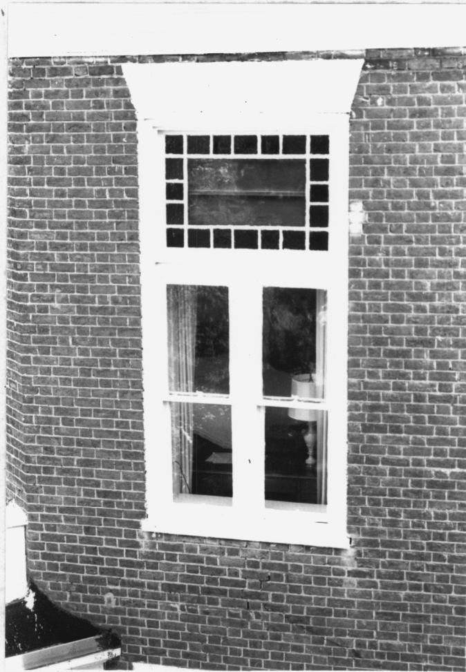
Fig. 11. Second story window of Preston Hall. Photograph by G. Hall
