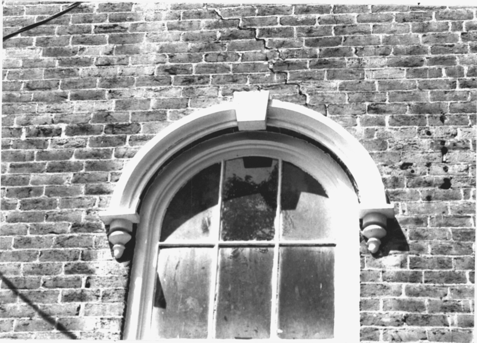
Fig. 16. East Hall - Window Detail Photograph by G. Hall
