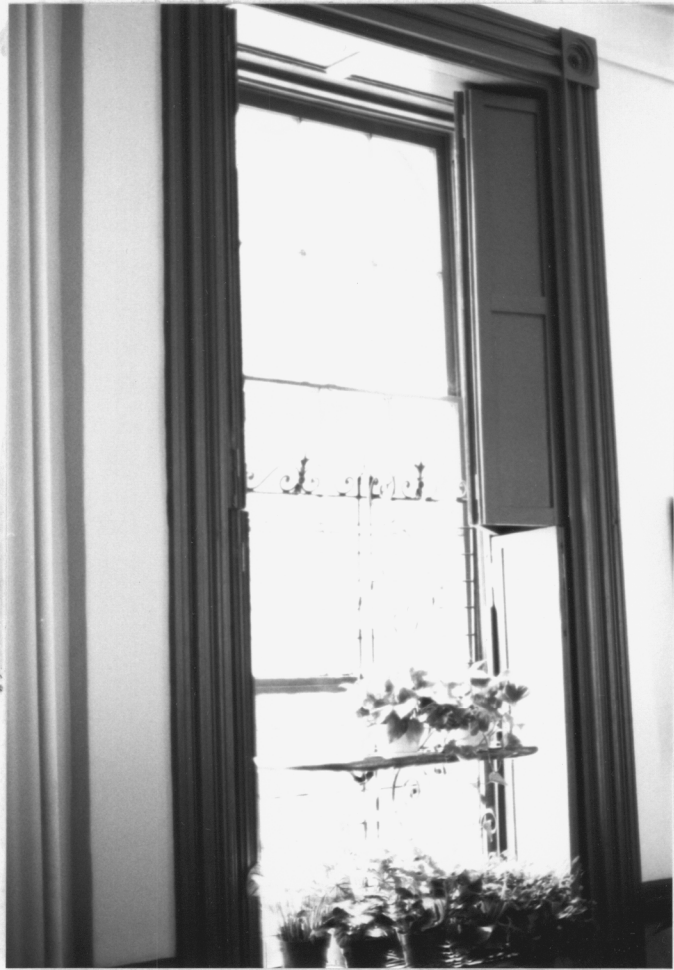
Fig. 8. Triple sash windows (8/8/12) with interior shutters on first floor of Preston Mansion Photograph by G. Hall
