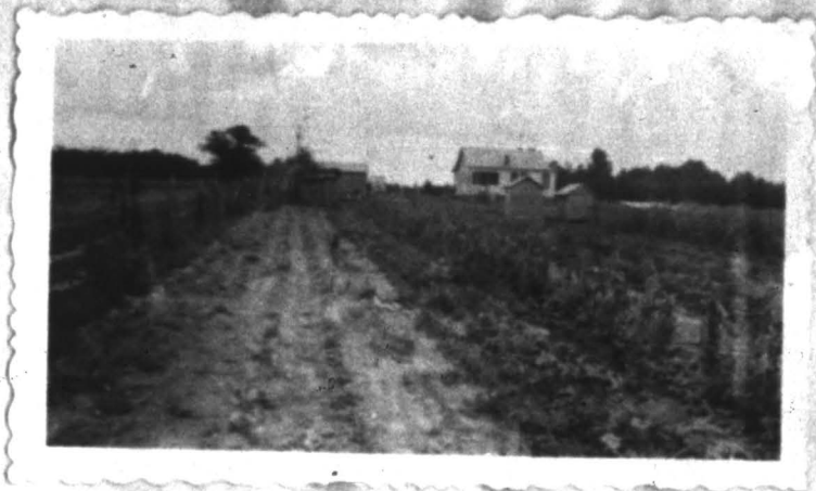
Road building demonstration leading to the home of James Tucker F. S. A. client, Greenville County
