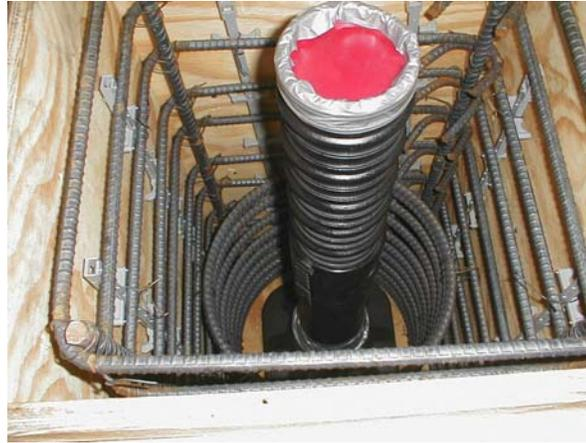
Fig. 1.5 Typical AASHTO Load Transfer Test Reinforcing. Source: VSL.
