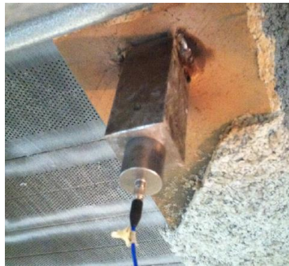
Figure 2. Accelerometer mount. Vertical, single-axis sensor shown. The mount is welded to a structural member with the fire retardant stripped to expose steel.
