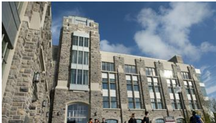
Figure 1. Goodwin Hall on the Virginia Tech campus.
