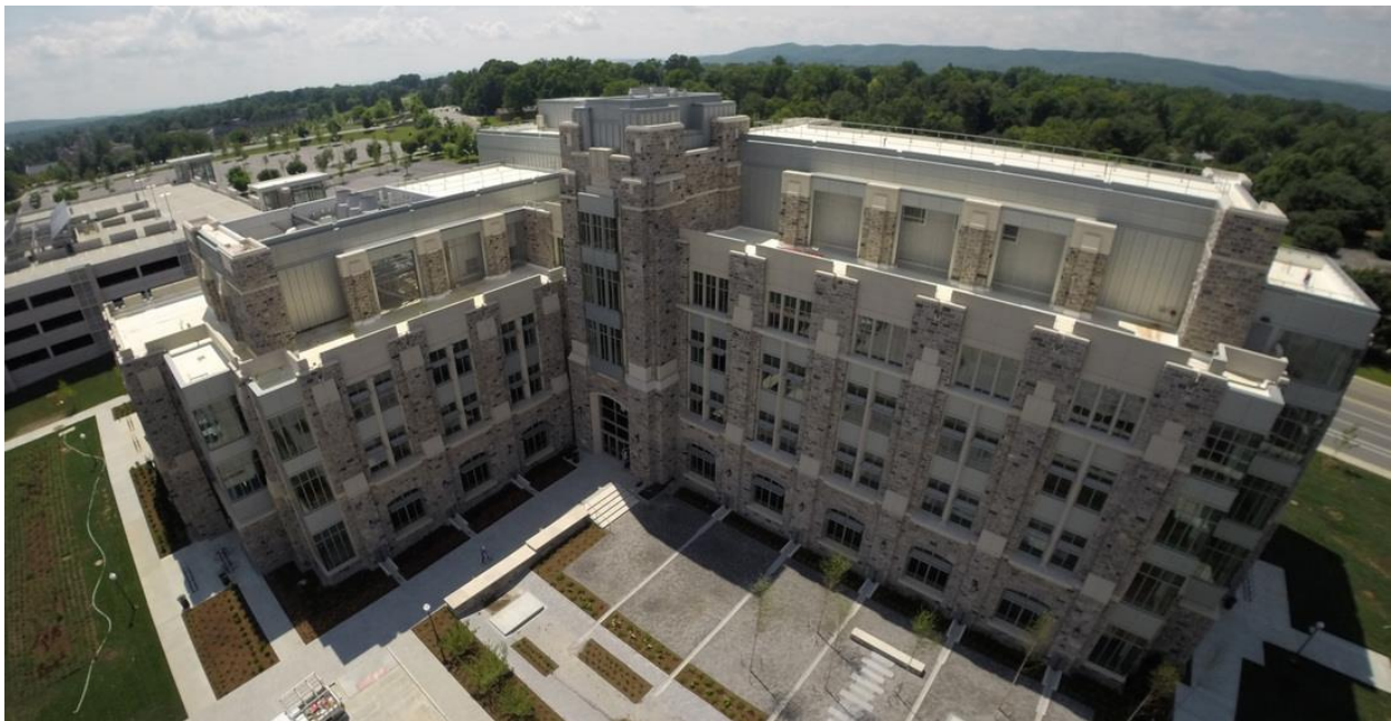
Figure 5. Aerial view of Goodwin Hall. Camera facing West.
