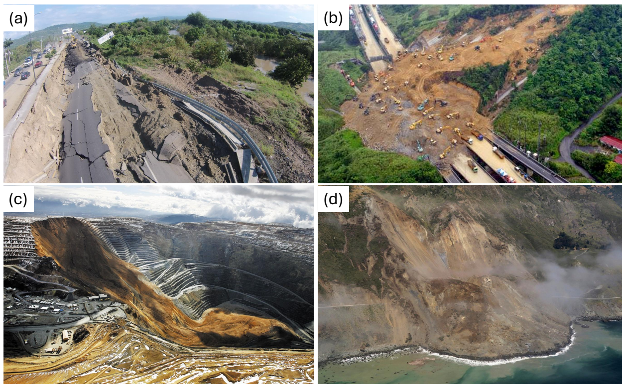
Figure 1.1: (a) Mejia embankment failure, 2016 M_w 7.8 Pederndales, Ecuador [4]; (b) Coseismic landslide disruption, 2014 M_w 5.0 Misca, Peru [5]; (c) Coseismic landslide in Bingham Canyon Mine, 2014 M_w 2.5 Salt Lake County, Utah [6]; (d) Coastal landslide, 2017 M_w 3.5 Big Sur, California [7]. Permission was granted from each author for the use of these photos in this dissertation.
