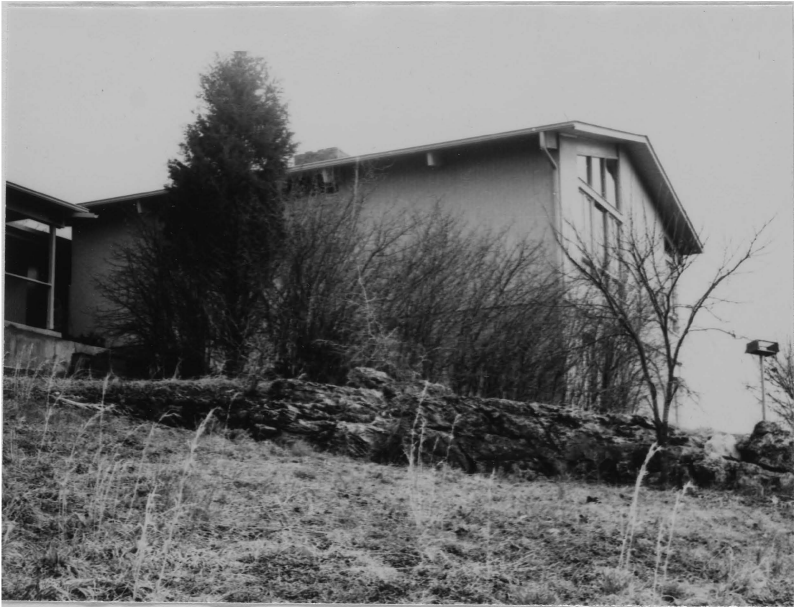
Natural stone outcrop beside a residence.
