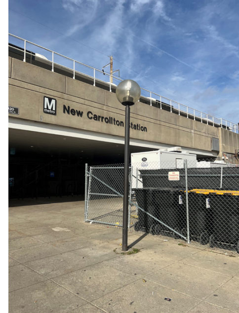
Eastside tunnel entrance facing north
