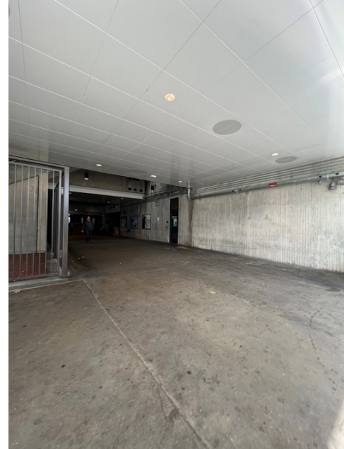
Tunnel facing northwest
