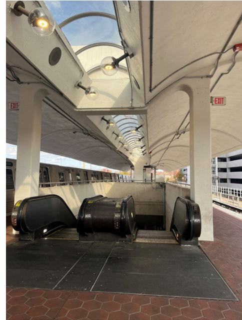
Metro platform facing northeast
