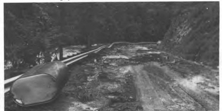
Someone's oil tank was washed downstream until it was lodged against a guardrail.
