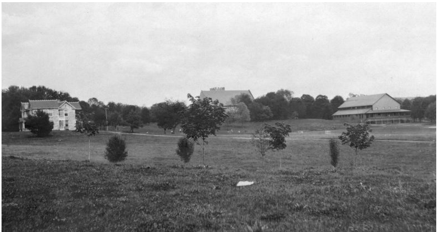
Figure 3. View of the Virginia Polytechnic Institute and State University campus in 1916, taken from unknown vantage point (Virginia Tech ImageBase, 2018c).
