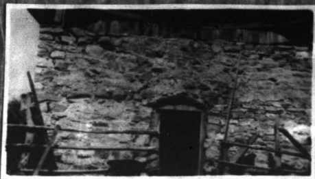
Potato Storage Mine Under Construction
