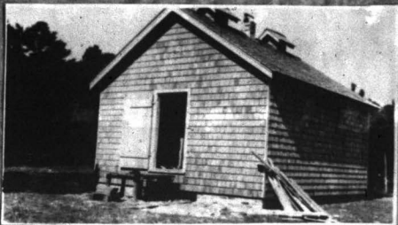
1000 sq. ft. House Constructed in 1934 - Princess Anne County
