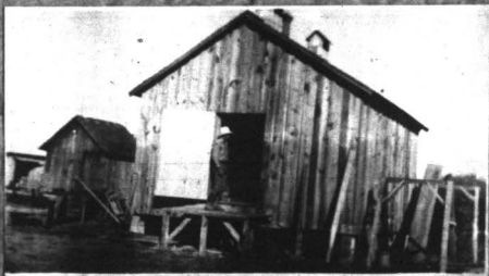
200 No. House Under Construction in Princess Anne County
