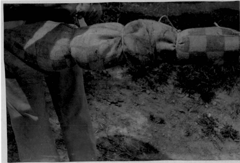
Figure 9. Securing sacks to core.
