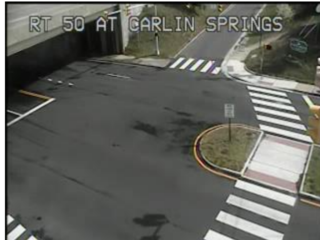
Figure 27. Camera view from the intersection between Carlin Springs Road and the Route 50 exit/entrance ramps.
