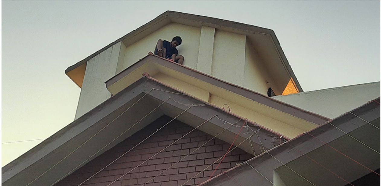
Figure 1.1: Harshal Pilania fixing lights on his house's roof
