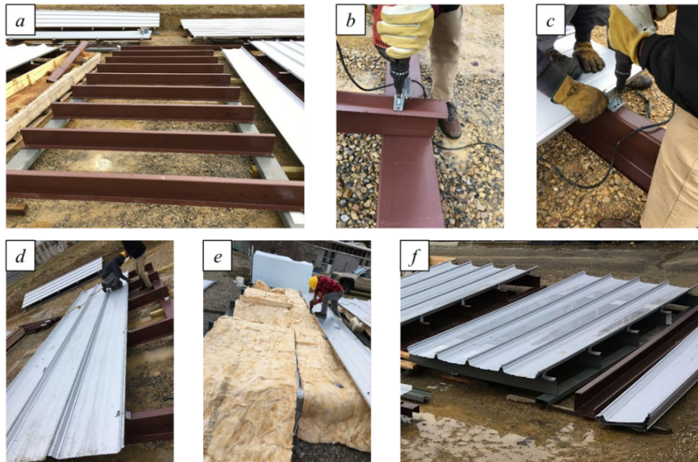
Figure 6-6 Specimen construction process
