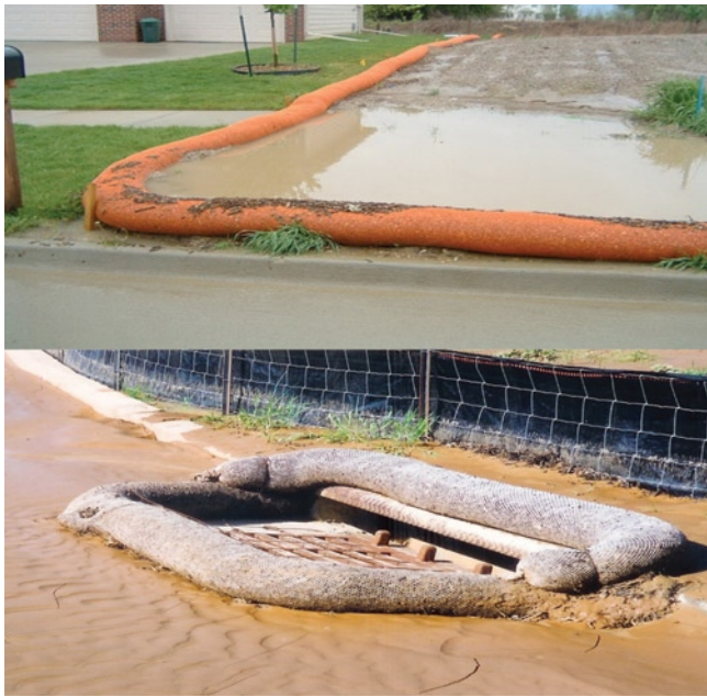
Figure 9.14. Compost in filter socks reduces runoff and protects stormwater quality.
