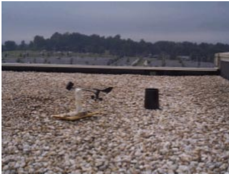
Figure 40: Weather monitoring system on rooftop of GBJ Student Center.
