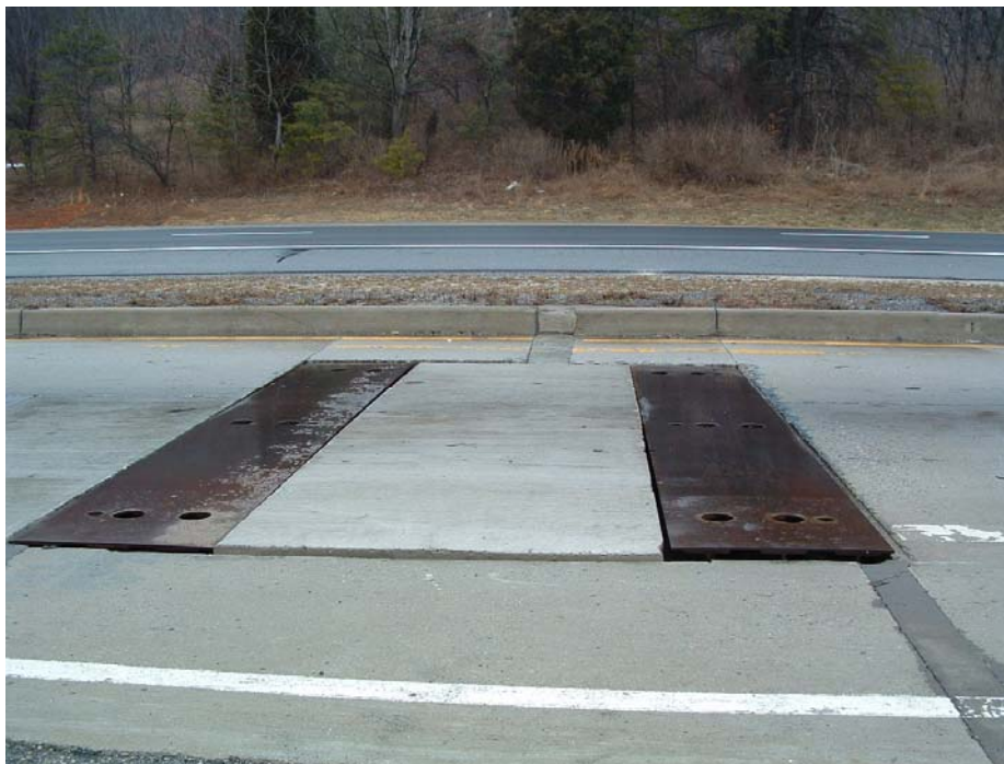
Figure 1.2: I-81 Weigh Station Slab
