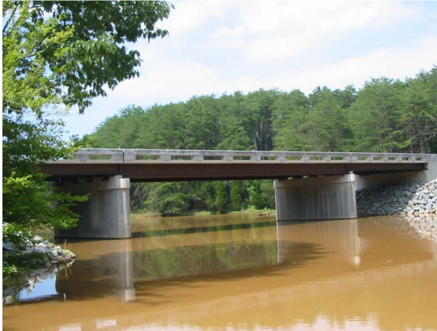
Figure 1.1: Route 668 Bridge Over Gills Creek
