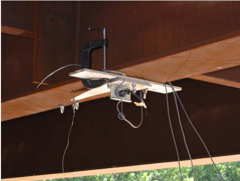
Figure 3.5: Deflectometer Clamped to Steel Girder
