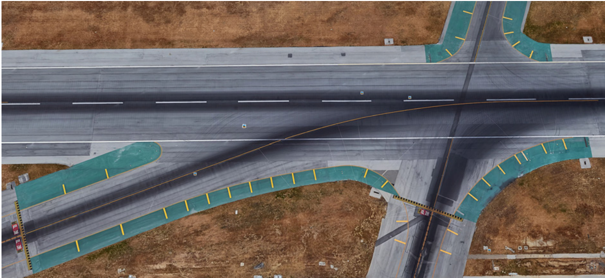
Figure 3.9: Image of Taxiway Centerline at San Francisco International Airport Runway 10L-28R. Source: Google Earth
