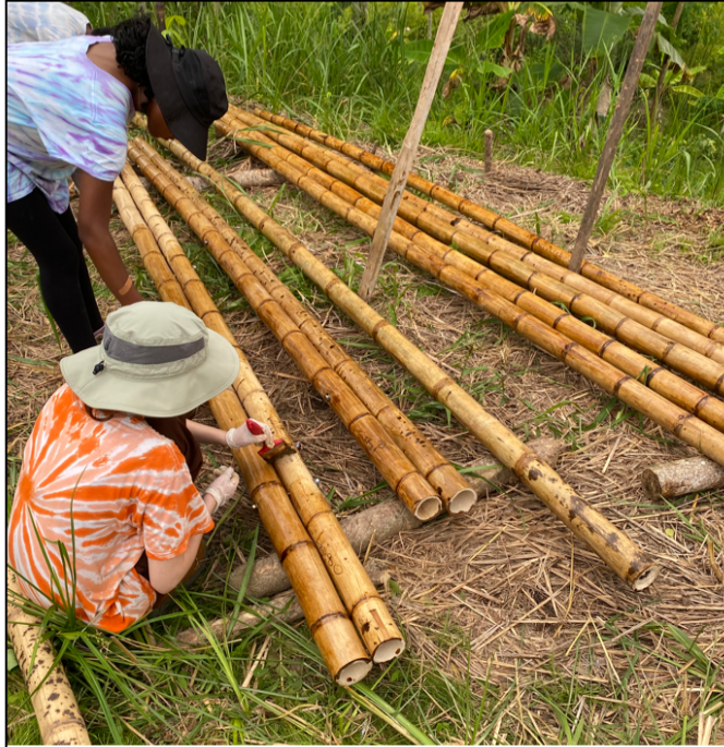
Figure B2. VT students apply a varnish to framing culms. Varnish helps seal and protect the bamboo from moisture and UV, while still displaying the natural grain patterns.
