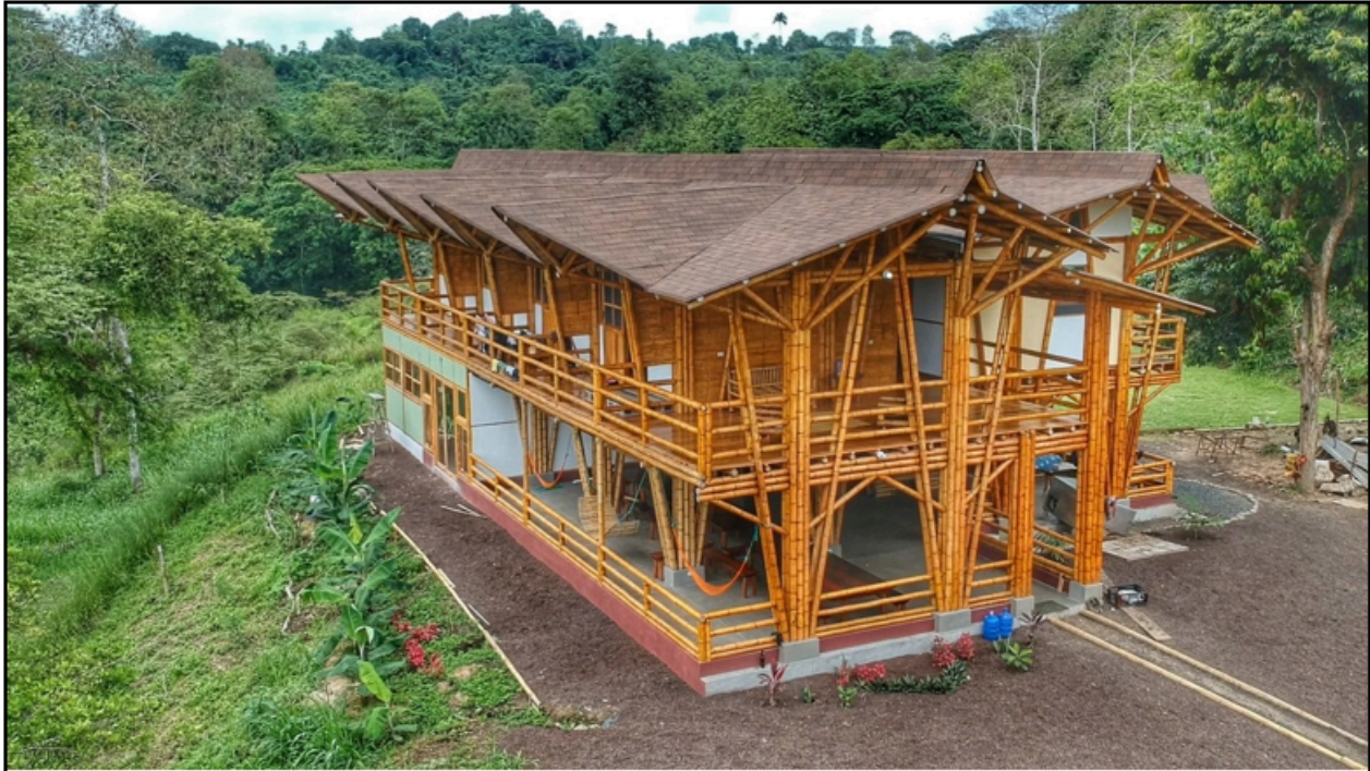
Figure 12. RFI headquarters at Los Arboleros Farm.
