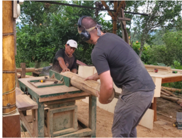
Figure 20. Processes. (top left) Installation of panels into the structure. (top right) Ripping round culms into strips for lathe. (middle left) Panel layout during gluing process. (middle right) Glue and top lathe applied to panel. (bottom) Panel transportation across the farm.
