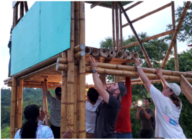
Figure 20. Processes. (top left) Installation of panels into the structure. (top right) Ripping round culms into strips for lathe. (middle left) Panel layout during gluing process. (middle right) Glue and top lathe applied to panel. (bottom) Panel transportation across the farm.
