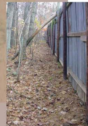
This section of the "Wall of Expression" is in good condition.
