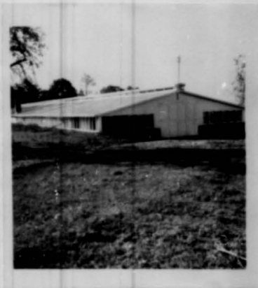
Commercial poultrymen are interested in better houses at less cost. This is the picture of a house that is 40' deep that has a driveway through the center and a ridge ventilator.
